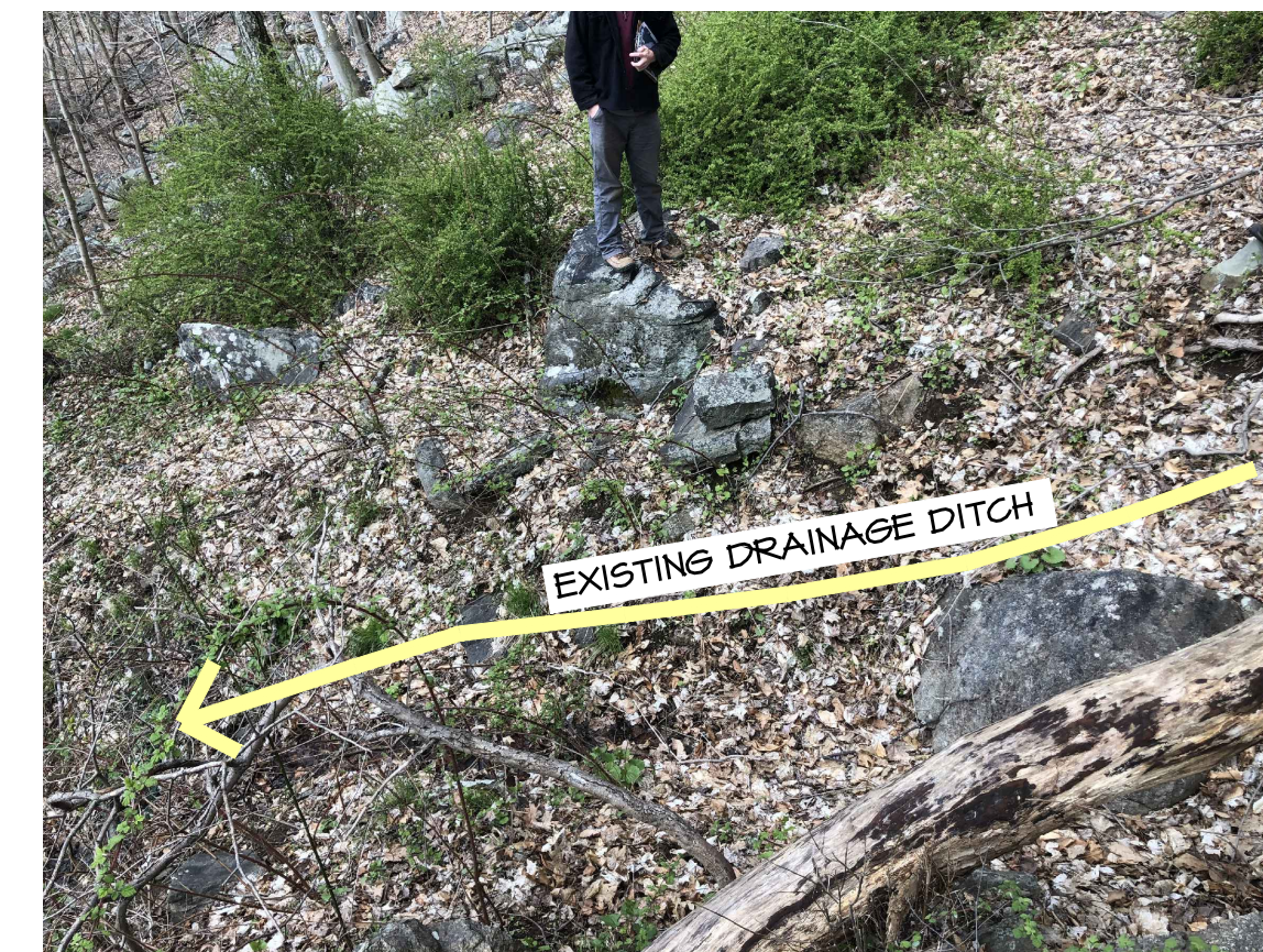
8 VIEW WEST OVER EX DRAINAGE CHANNEL AND OPPOSING ROCK OUTCROPS. GABION BASKETS SHALL BE INSTALLED BETWEEN THE OUTCROPS TO CREATE A SEDIMENT SUMP IN THE DRAINAGE CHANNEL TO CAPTURE SUSPENDED SEDIMENT FOR ROUTINE REMOVAL BEFORE IT CAN ENTER THE LAKE. NOTE PRESENCE OF INVASIVE JAP. BARBARY TO BE REMOVED
