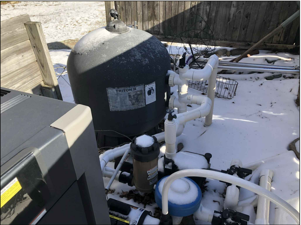
VIEW TO POOL EQUIPMENT AREA AND OUT DATED SAND FILTER. A NEW CARTRIDGE FILTER WILL BE PROPOSED TO ELIMINATE THE NEED TO BACK WASH THE SAND FILTER.
