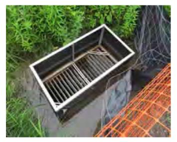
The drainage area shall be limited to 1 acre at the drain inlet. All inserts will be installed and anchored in accordance with the manufacturers recommendations and design details. The fabric portion of the structure will equal or exceed the performance standard for the silt fence fabric. The inserts will be installed to preserve a minimum of 50 percent of the open, unobstructed design flow area of the storm drain inlet opening to maintain capacity for storm events.
